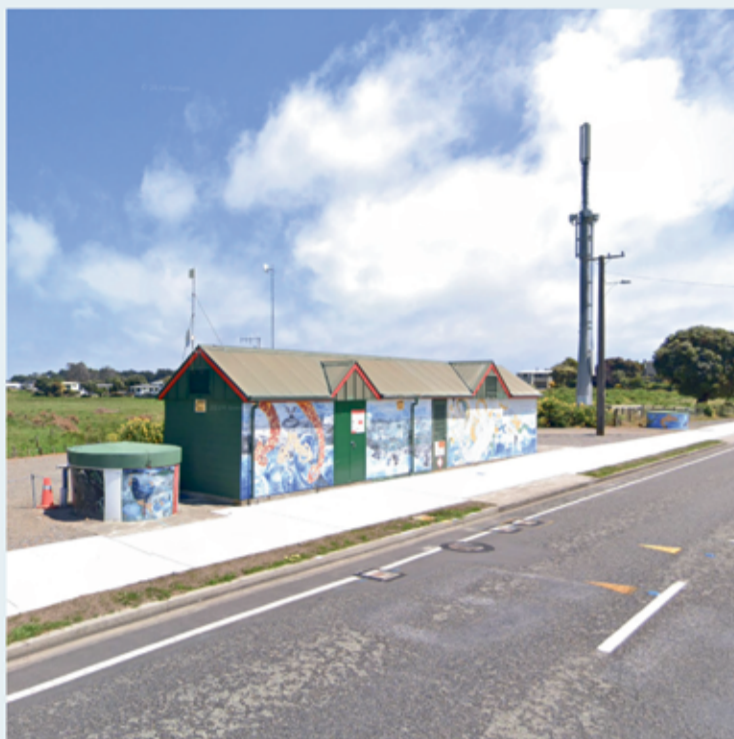
Tasman Road bore drilling location
